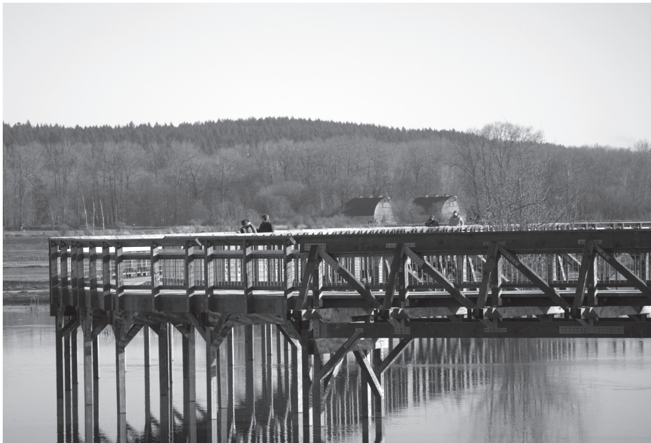
New boardwalk at Nisqually Delta. Photo by Judy Murphy. February 2011.
